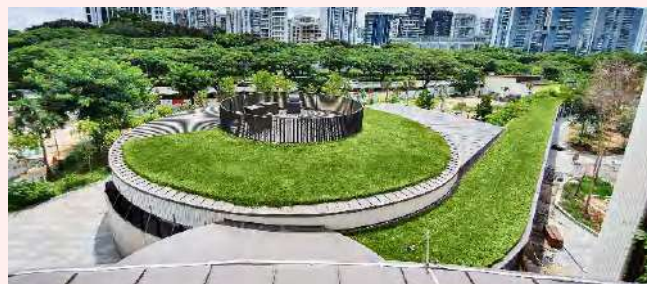
Pictured: Lysaght® Green Roof Solution installed on a restaurant within the East Coast Park in Singapore.
